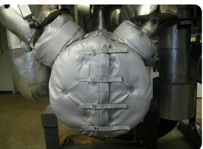
Recommended Service/Use: valves, flanges, expansion joints, Y-strainers, heat exchangers, pumps, turbines, tanks, PRV stations and boilers typically found in central plants, mechanical rooms, manholes, vaults, tunnels and other confined spaces.
