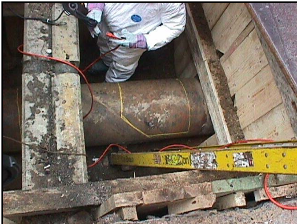
The 18-inch outer steel casing is marked prior to cutting/grinding.
